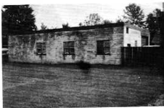
The Garage Alma Street
